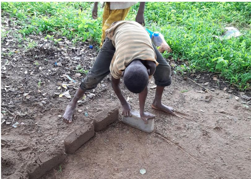
*Moulding and laying air-dried mud bricks*
